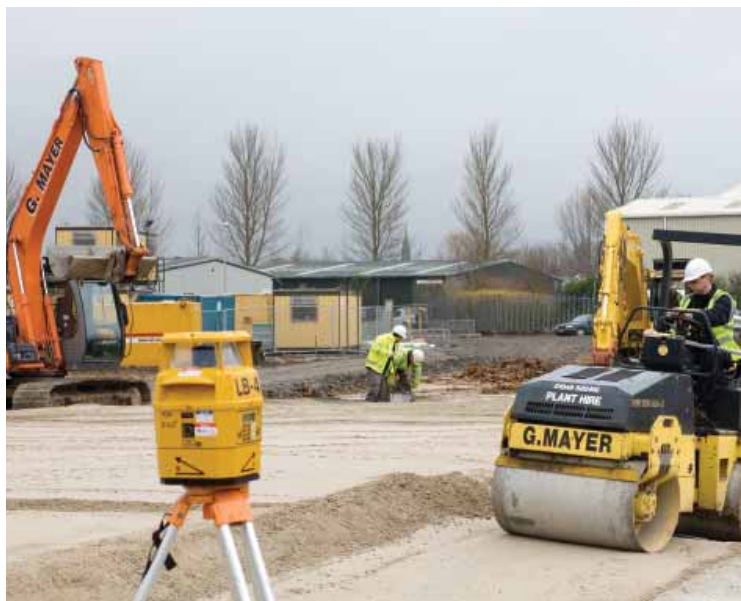
Winsford Household Waste Recycling Centre under construction
